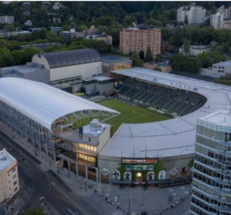
5. PROVIDENCE PARK USA - BY TETRA TECH
