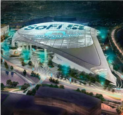
3. SOFI STADIUM USA - BY TETRA TECH
