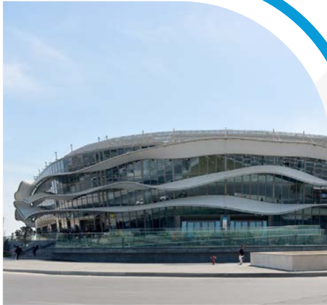
4. BAKU GYMNASICS ARENA AZERBAIJAN - BY ROBERT BIRD GROUP
