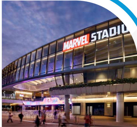
MARVEL STADIUM REDEVELOPMENT MELBOURNE, VIC, AUSTRALIA - BY NDY
