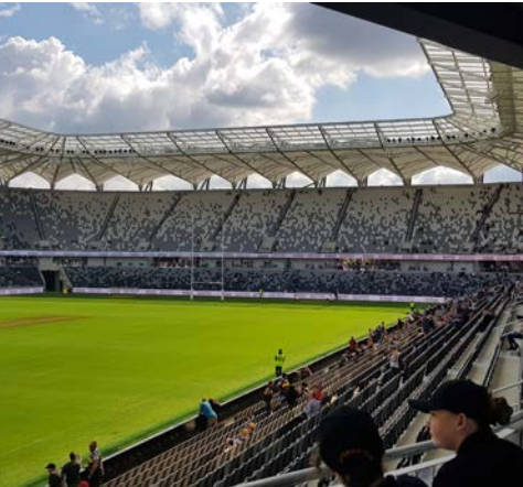
WESTERN SYDNEY STADIUM SYDNEY, NEW SOUTH WALES - BY ROBERT BIRD GROUP
