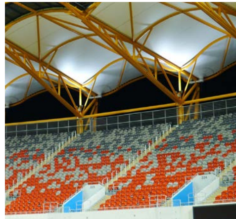
PEOPLE FIRST STADIUM (CARRARA STADIUM) CARRERA, QUEENSLAND - BY NDY
