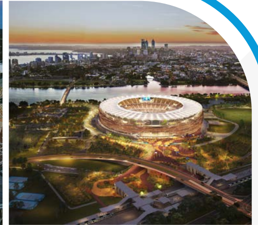
OPTUS STADIUM PERTH, WESTERN AUSTRALIA
