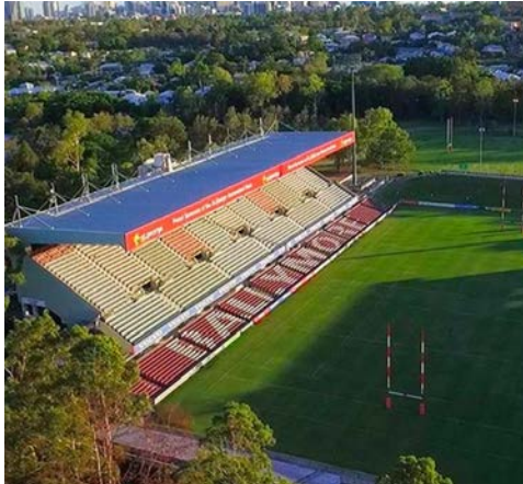
BALLYMORE EASTERN GRANDSTAND BRISBANE, QUEENSLAND - BY ROBERT BIRD GROUP
